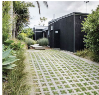
DRIVEWAY AND ENTRY PATH PAVING PERMEABLE GRASS CRETE, CONCRETE BLOCKS WITH SAND AND COUGH GRASS BETWEEN
