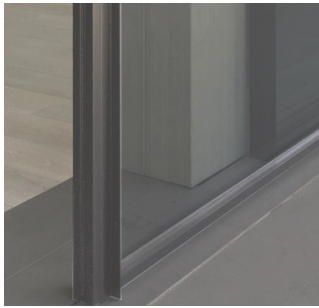
CLEAR GLAZING WITH CHARCOAL ANODIZED ALUMINIUM FRAMES W-01 WINDOWS AND DOORS
